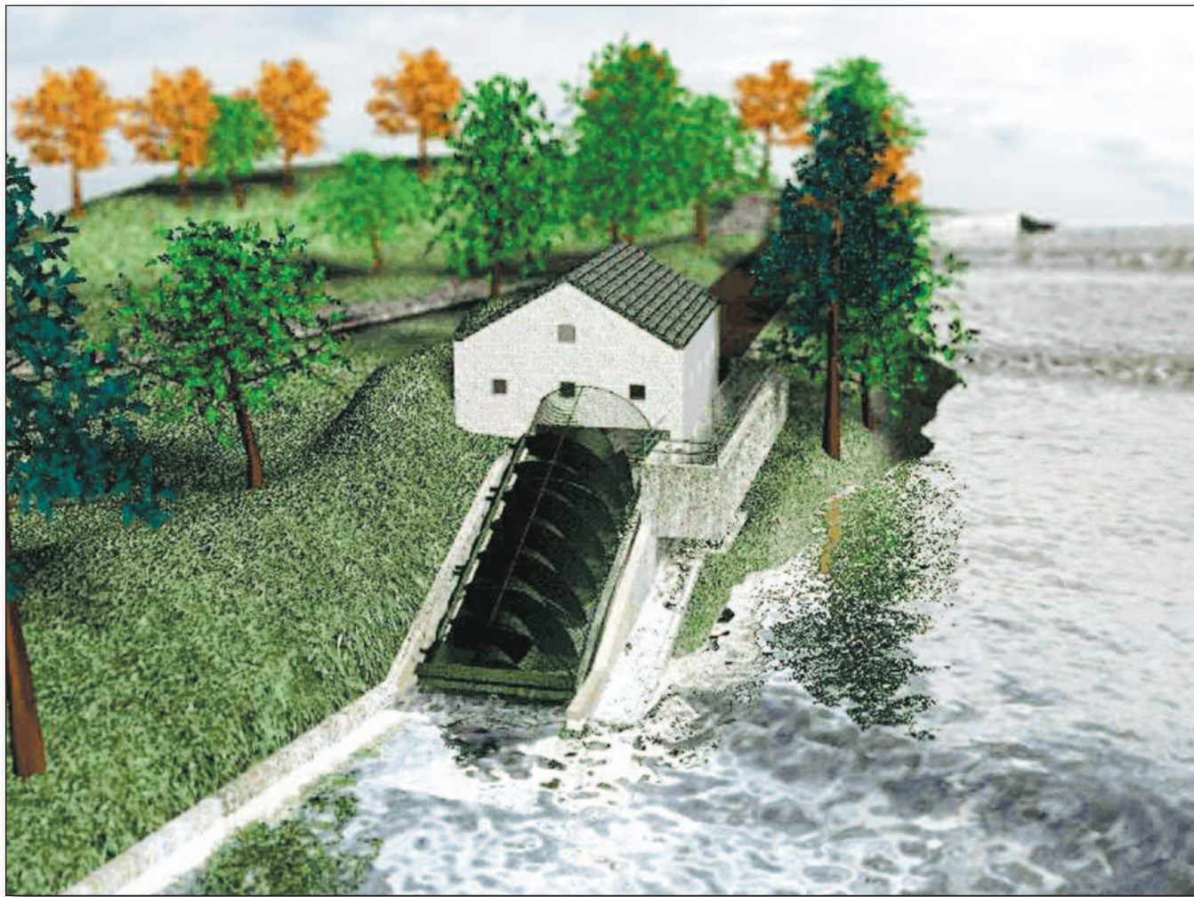
■ LEFT: An artist's impression of the Archimedean screw hydro turbine on Camowen River in Omagh, which will generate sufficient power to meet the needs of the Omagh Leisure Complex.
